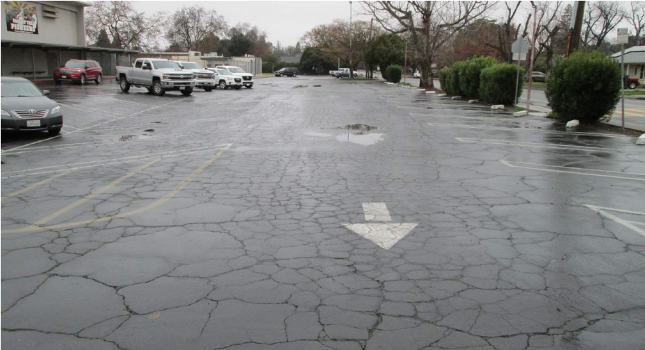
Cracked Asphalt at parking and play areas
