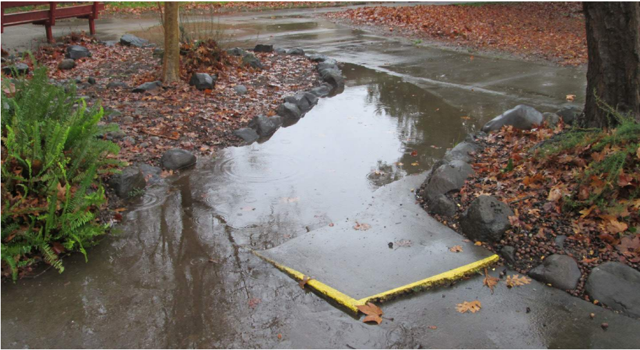
Ponding of water around site. More adequate drainage needed
